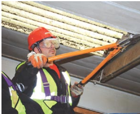
Removing hook bolts from existing sheet
