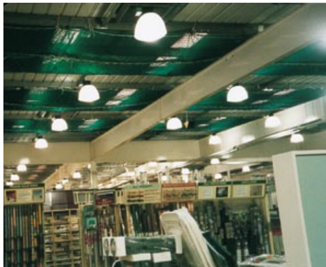
Safety netting used to provide protection for roof lights during minor roof works
